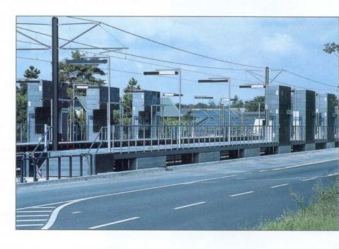
For the new D-Süd urban railway line from the Hanover city centre to the EXPO site, architects Günther and Martin Despang developed a modular concept of 13 elevated railway platforms and waiting cabins suspended on a filigree steel base construction. The platforms at the 'Pressehaus' station and the cubic waiting blocks with their numerous integrated functions are clad in basaltic lava.
