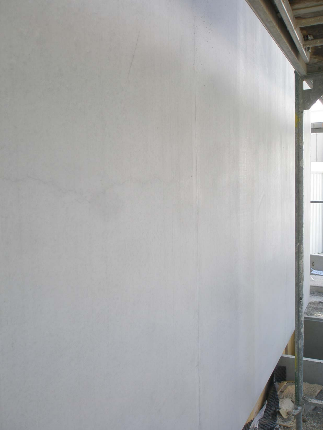
concrete as smooth as the required stucco / plaster
