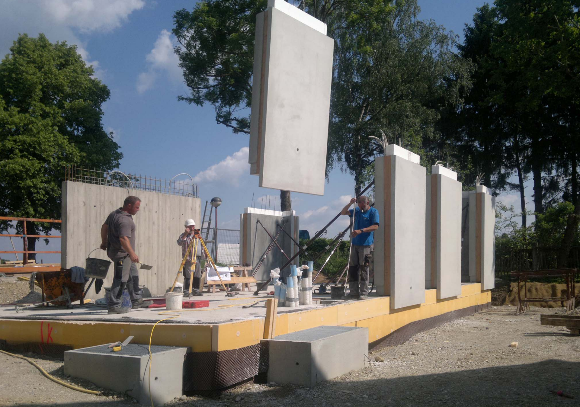
adapting for the 21st century with prefabricated insulated sandwich ( tilt up ) panels
