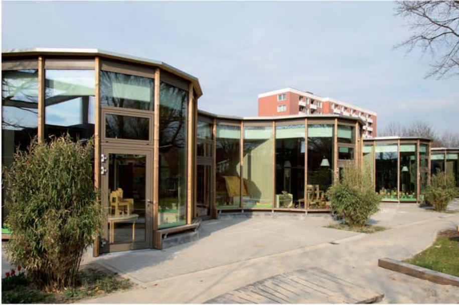
↑ | Exterior view ← | Detail, façade
