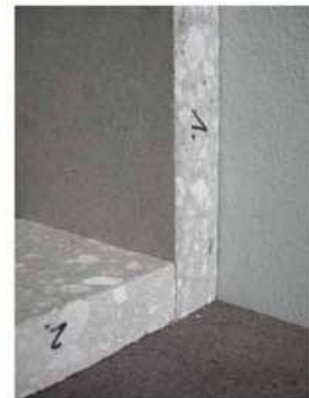
concrete slab and floor
