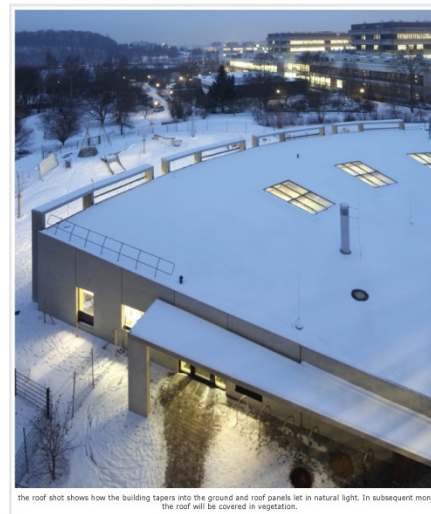
the roof shot shows how the building tapers into the ground and roof panels let in natural light. In subsequent months the roof will be covered in vegetation.
